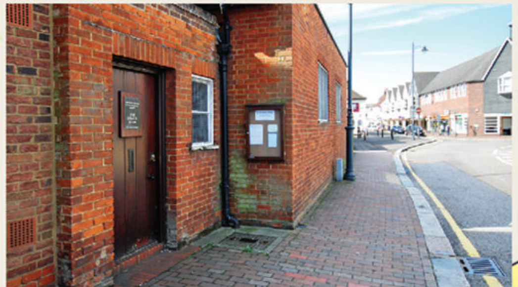
Friends' Meeting House Entrance, 50 Railway Street
