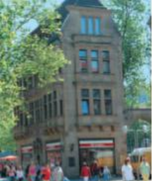
6 Vehoff-Haus Vehoff House
